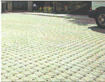
10,000 square feet of Unilock Ecolock paver
