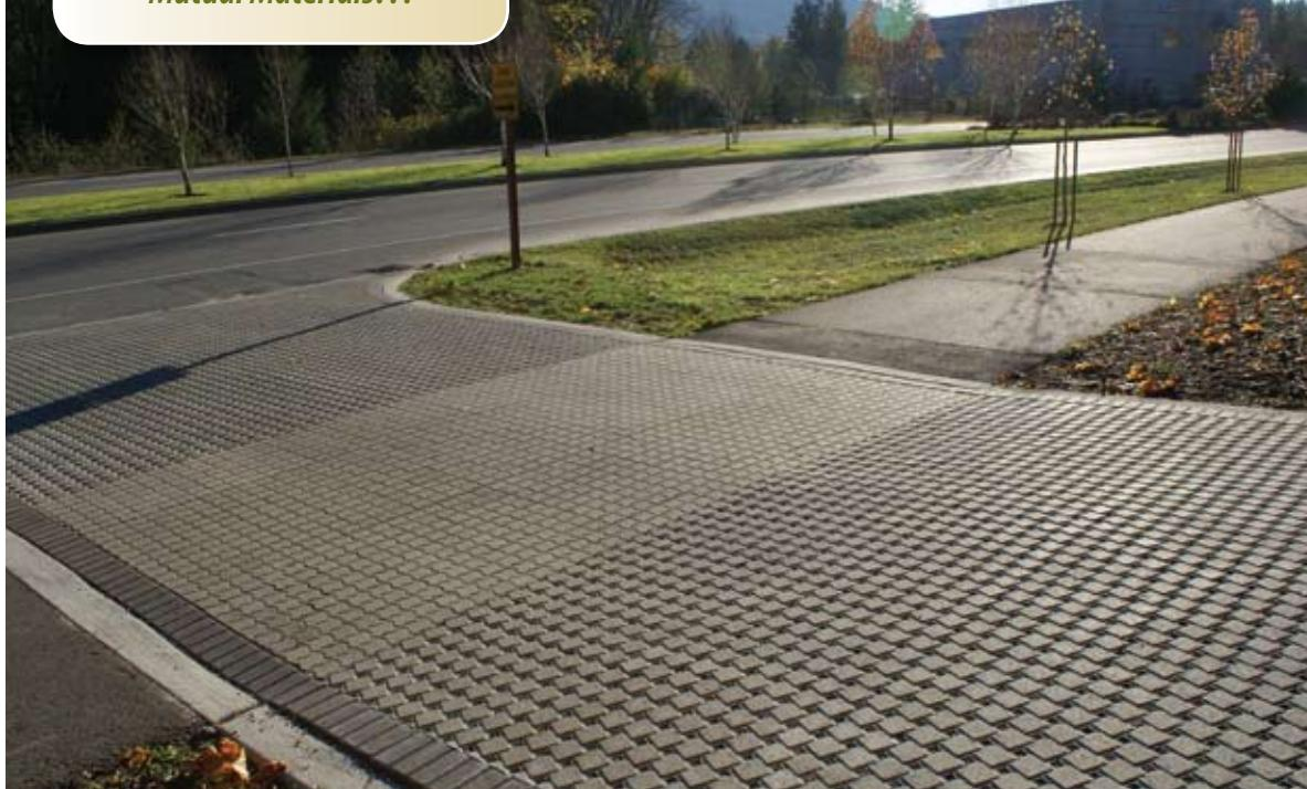
Permeable pavers can sustain heavy apparatus loading.
