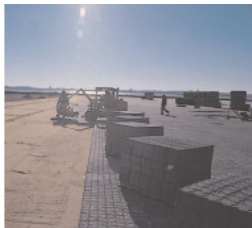
Like the past projects, recent construction of paving at Seagirt used mechanical equipment placing concrete pavers manufactured and stacked in the final laying pattern.
