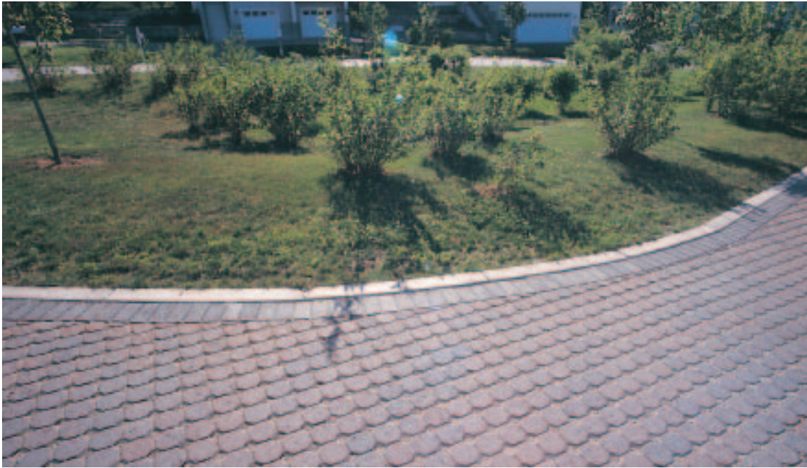
Figure 4. A rain garden in the center of the cul-de-sac soaks up runoff in a space that would otherwise be paved with an impervious surface.
