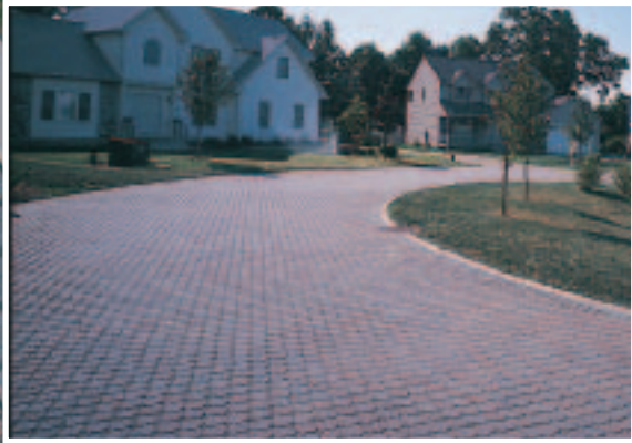
Runoff is being monitored from over 15,000 sf (1500 m 2 ) of permeable interlocking concrete pavement in the road and driveways of the Glen Book Green Subdivision in Waterford, Connecticut.
