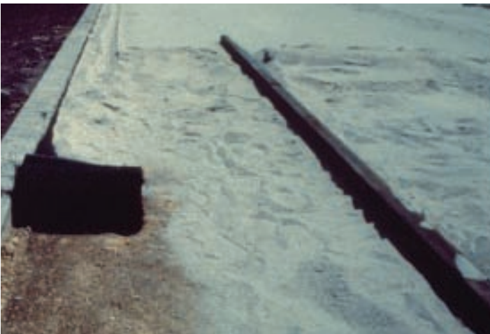
Figure 6. A strip of geotextile contains bedding sand against a curb.
