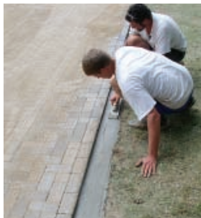
Figure 2. Troweled concrete detail and installation. This edge restraint is intended for mild climates and residential uses only.
