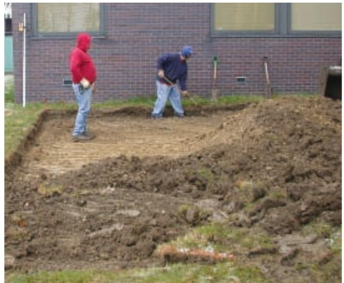
Figure 5. A clean excavation cut in the soil may need some touching up with a shovel to create perpendicular sides.
