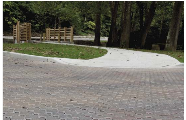
Figure 2. Cascades Creek bisects two permeable interlocking concrete pavement parking lots in the park joined by this foot bridge. The filtering action of the permeable base protects the lovely Creek which passes through waterfalls.
