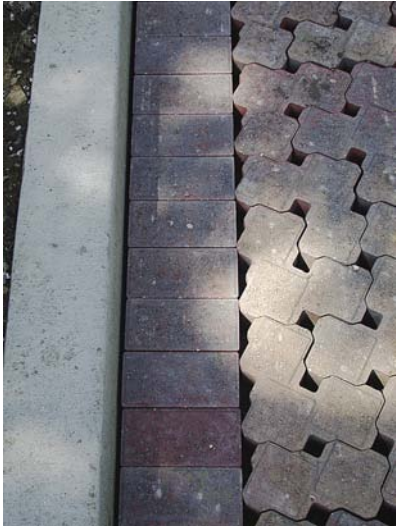
Figure 5. A soldier course against the cast-in-place concrete curb facilitates mechanical placement by providing space for machine clamp to insert paver layers without interfering with the curb.
