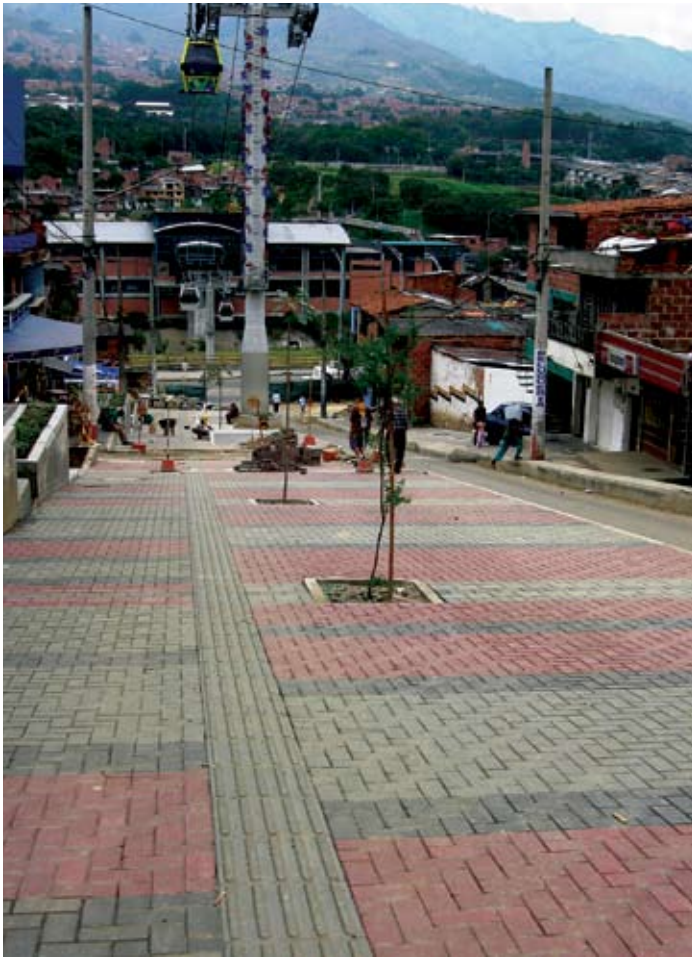
Figure 3. Redevelopment of popular neighborhood in Medellín, Columbia included a 14% slope for the sidewalk and adjacent street.
