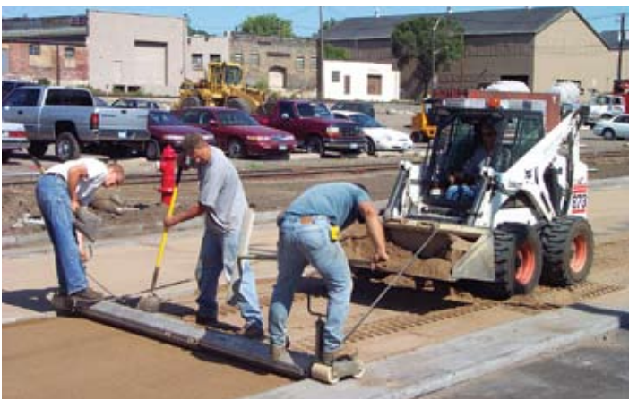
Figure 6. Mechanical screeding is the most efficient method of bedding sand installation. In the largest projects, a laser guided asphalt spreader (right) can be used to accurately screed bedding sand.
