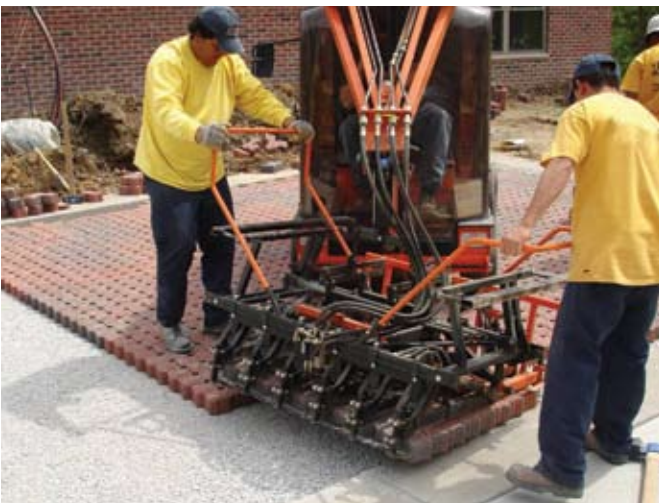
Figure 6 and 7. Mechanical installation equipment places ready-made layers of the concrete pavers. The equipment generally reduces paver installation time by 50% to 70% compared to manual installation.
