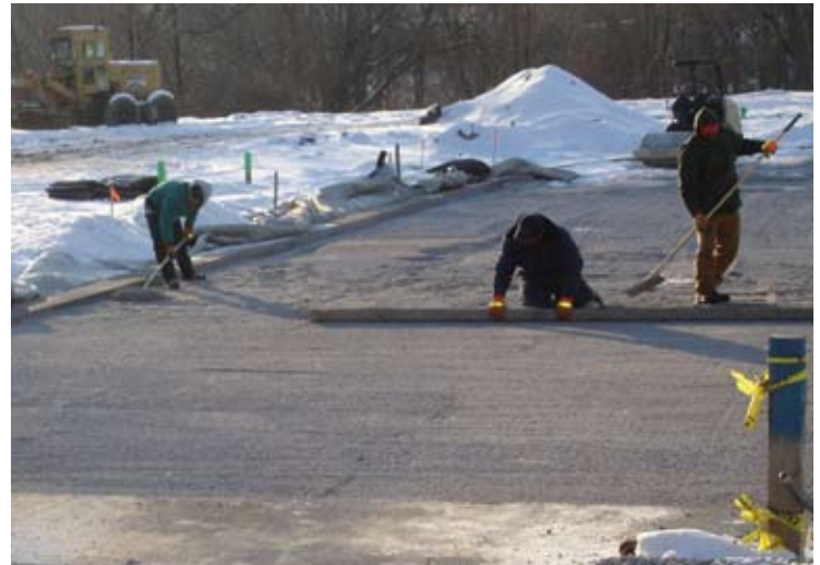
Figures 3 and 4. Compaction equipment completes the base surface prior to placing the bedding layer and screeding it smooth to receive the permeable pavers.
