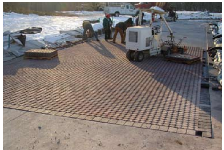
Figure 6 and 7. Mechanical installation equipment places ready-made layers of the concrete pavers. The equipment generally reduces paver installation time by 50% to 70% compared to manual installation.
