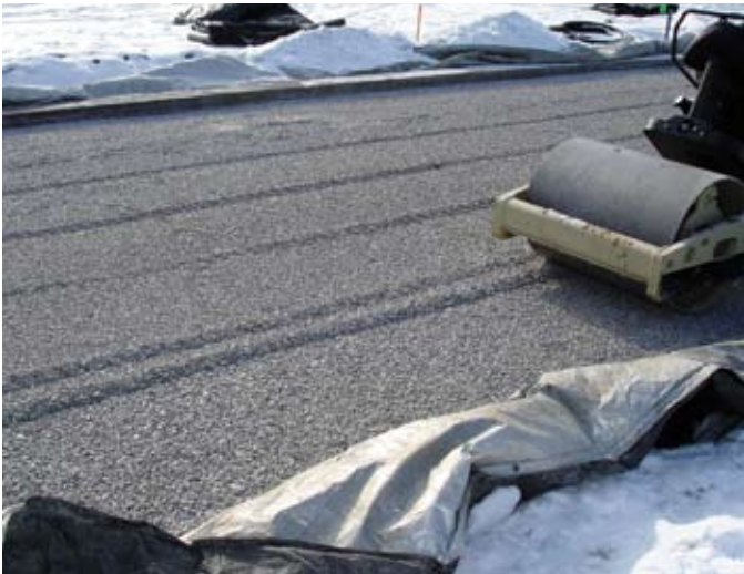
Figures 3 and 4. Compaction equipment completes the base surface prior to placing the bedding layer and screeding it smooth to receive the permeable pavers.
