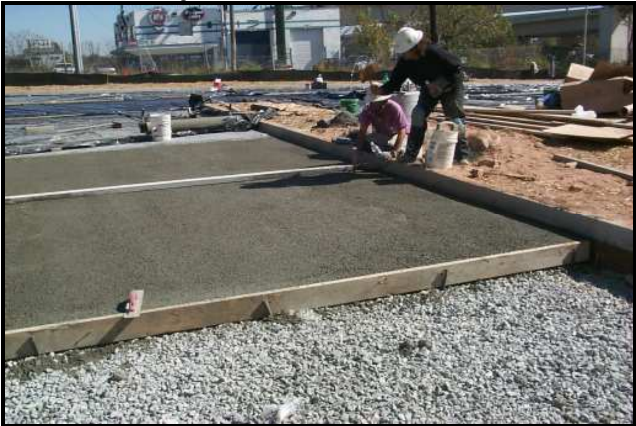
Figure 4-54. Porous Pavement Installation
