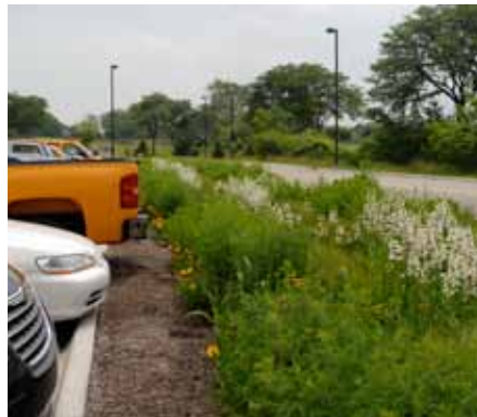
Parking Lot Bioswale
