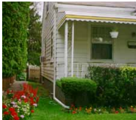
Downspout Disconnection
