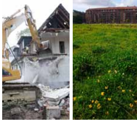
Vacant Home Demolition/Revegetation
