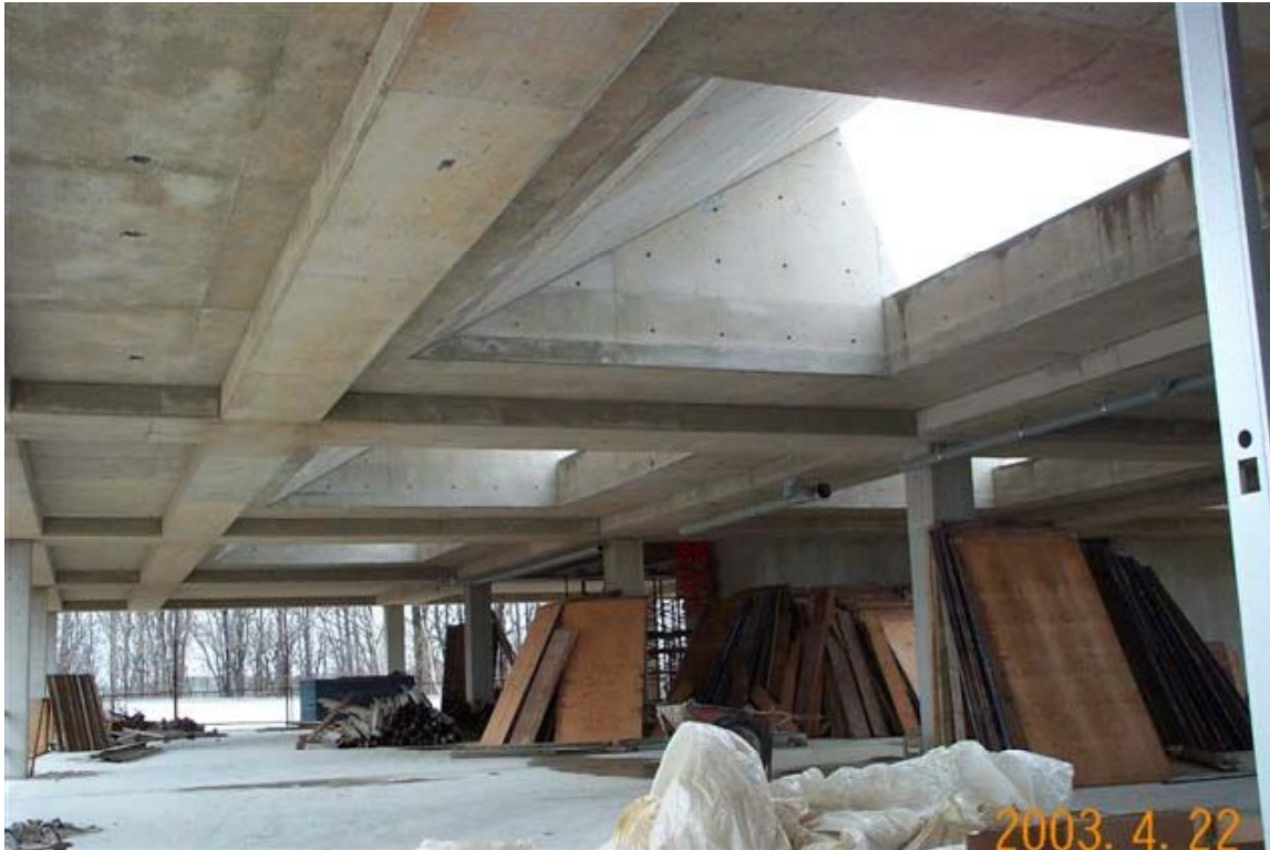
Figure 1. Skylights for daylighting and solar collector mounting. Exposed concrete structure.
