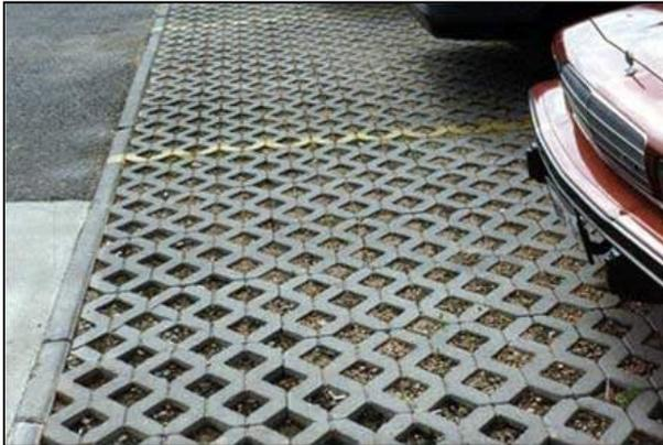
**Description:** A pavement surface composed of structural units with void areas that are filled with pervious materials such as sand or grass turf. Porous pavers are installed over a gravel base course that provides storage as runoff infiltrates through the porous paver system into underlying permeable soils.
