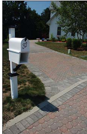
Gaps in permeable concrete pavers draw rainwater into the ground, minimizing runoff. (By Bruce K. Ferguson)
