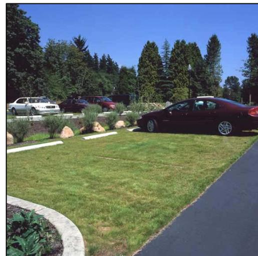
Permeable Pavement Layer – This layer consists of a porous mixture of concrete or asphalt or a modular pavement grid of plastic, concrete, or brick and an aggregate or a vegetation medium. This layer is usually 2 to 4 inches deep depending on required bearing strength, pavement design requirements, and manufacturer's specifications.
