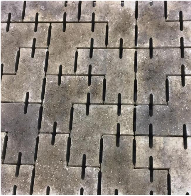
Figure 2: Pavement constructed from two L-shaped PICP blocks with cupules of two different lengths aligned in the direction of sweeper travel. Real cupules have rounded edges; cupule width is 12.5mm, block joints are typically 2 mm wide.
