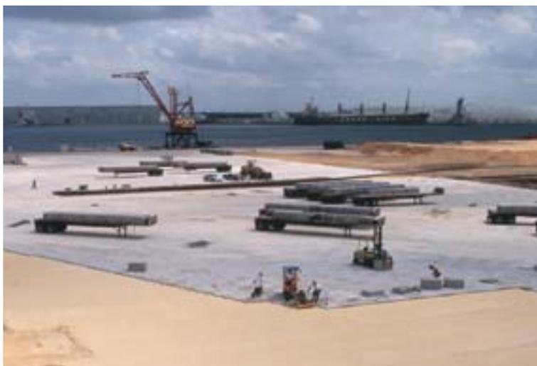
From 8,000 to 12,000 square feet of UNI-Anchorlock® pavers was installed per day using mechanized paver placement and sand screeding equipment
